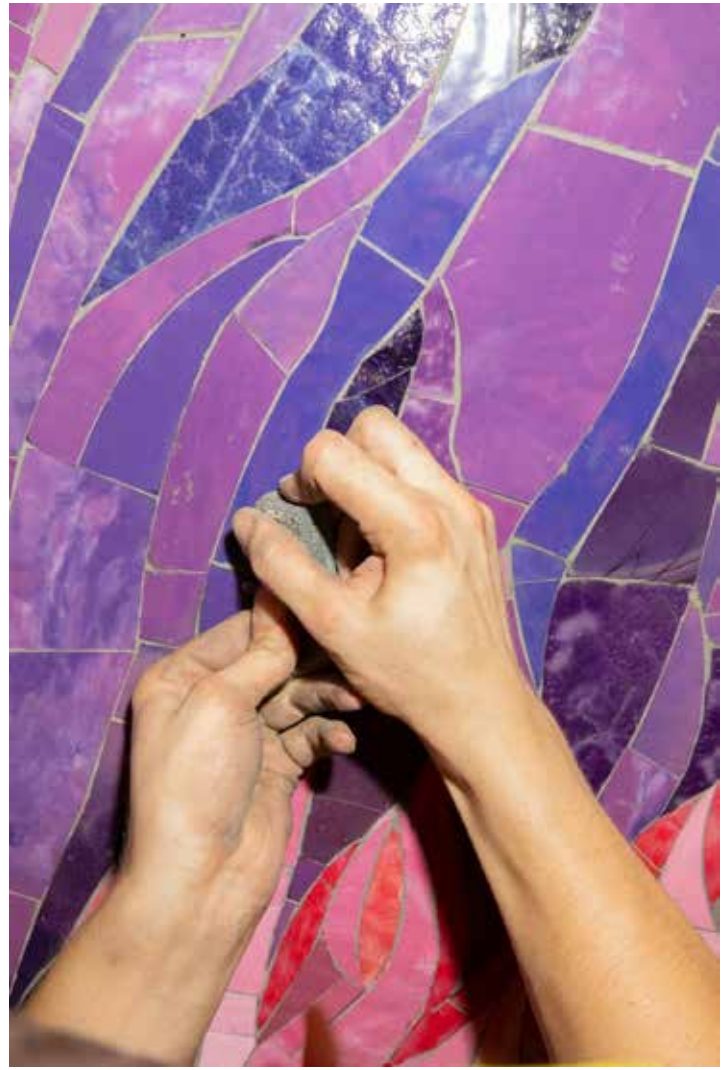
A worker uses a file to smooth rough edges of the mosaic. Sinna Nasser for The New York Times
